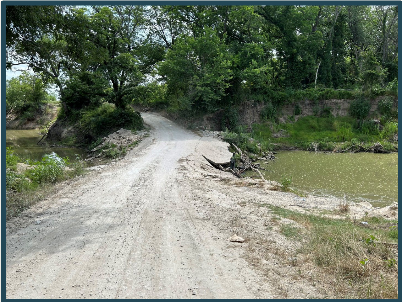
Figure 25. Low water crossing on Straws Mill Road
