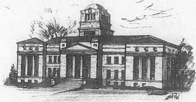
Navarre County Courthouse
