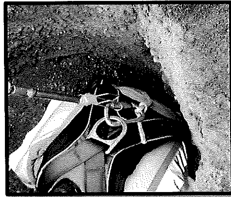
Figure 5. When the carabiner has engaged the D-ring, the pole shall be pulled away from the D-ring (quickly), and the rescue device will be secured.
