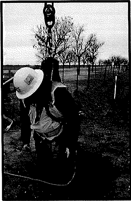
Figure 6. When determined safe to proceed, the employee will be hoisted to the surface using the rescue system.
