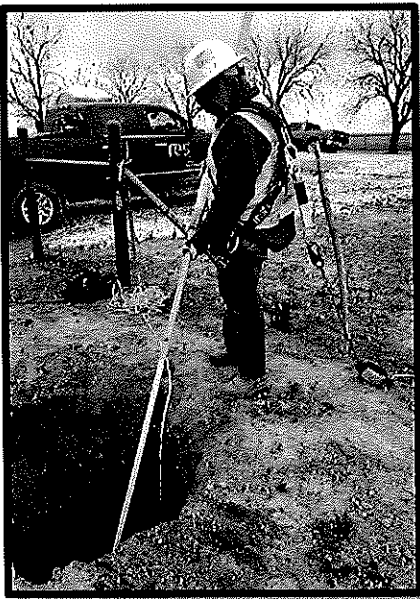
Figure 3. The rope/carabiner will be lowered to the employee utilizing the rescue remote connection pole.
