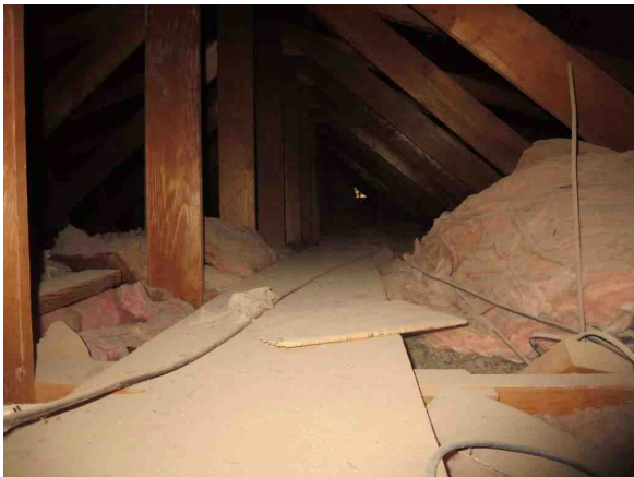
Attic View Rolled-in Insulation
