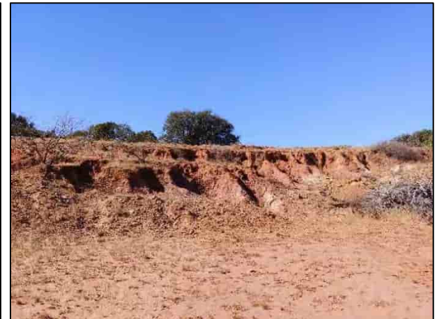
About 200 ft upstream of crest
