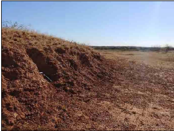
At right end of embankment, looking downstream
