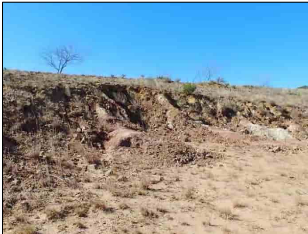
About 50 ft upstream of crest
