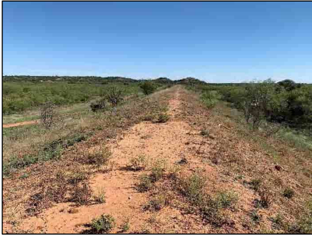
Crown of dam and embankments (10/2020)
