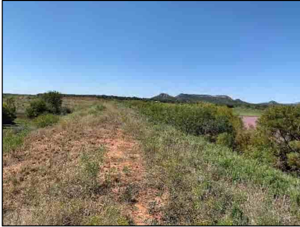
Crest and embankments
