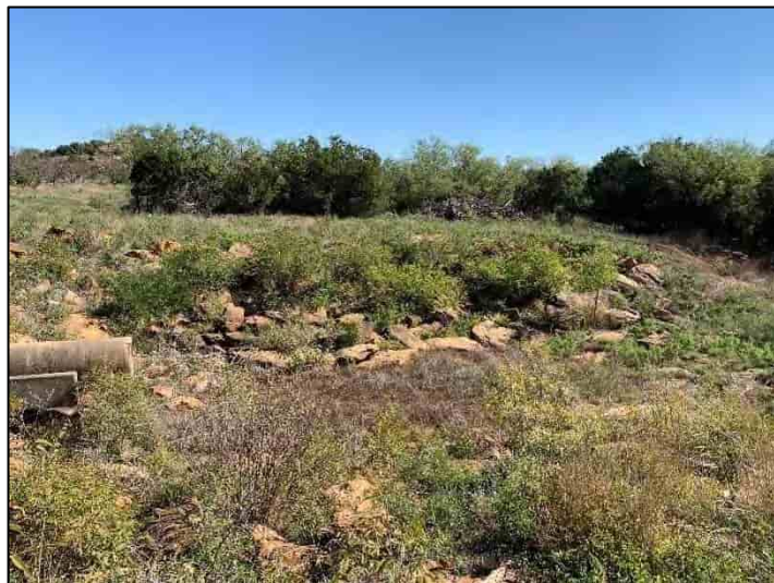
Outlet pipe and plunge pool (10/2020)
