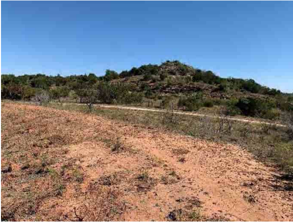
Auxiliary spillway control section (10/2020)
