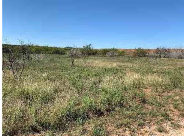
Auxiliary spillway exit section (10/2020)
