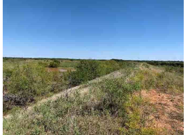
Crest and upstream embankment
