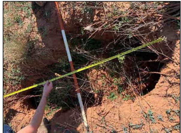
Large hole resulting from longitudinal cracking. (10/2020)
